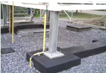
Container Grounding System
