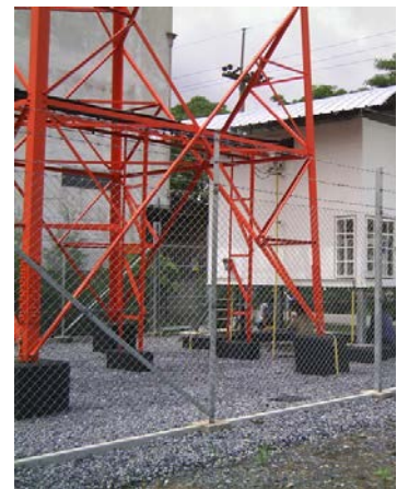
Fence Installati on Comple ted
